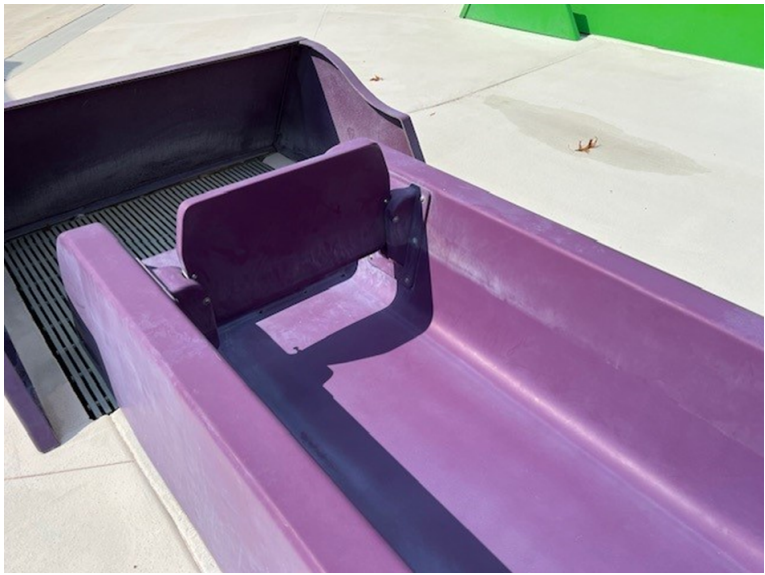
Reduction of scale on Tembo Slide AFTER using PoolMoss
