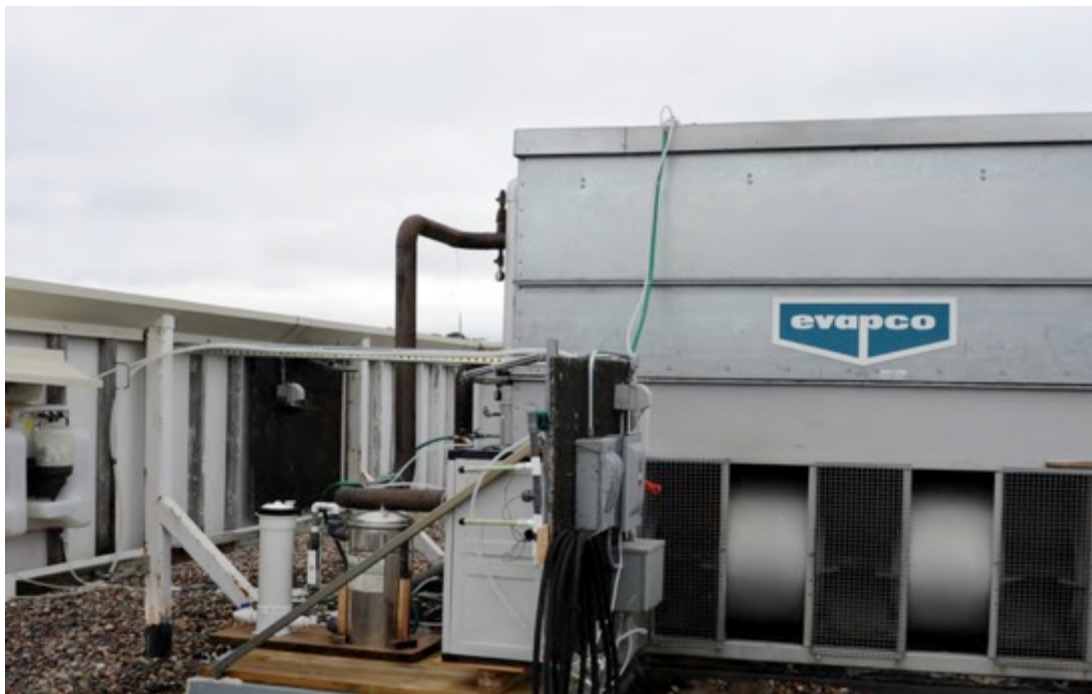
Sphagnum moss delivery system used on three different facilities. Stainless steel tank contains the Sphagnum moss, white PVC cylinder is a filter and two LPR probes are in line.
