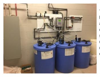
Take for example the chemical feed setup shown here. While it is doing a great job at reducing corrosion and controlling microbiological contamination, it is complicated. A large footprint is required for the system, and most people working in the facility do not understand how it operates. For decades this was the only solution to extending the life of industrial cooling equipment.
