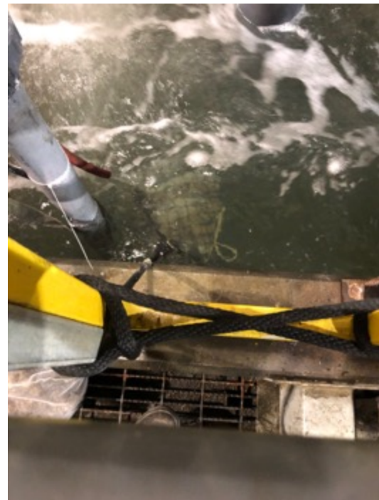
Picture taken on December 7 th of cooling tower sump with ProMoss™. The cage with the ProMoss™ in it can be seen and is 3 feet below the water surface. Notice the clarity of the water.
