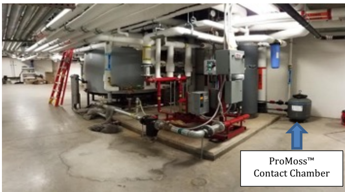
Rain Water collected from the roof is used as “gray water” for flushing toilets, thus reducing the demand for fresh city water.
