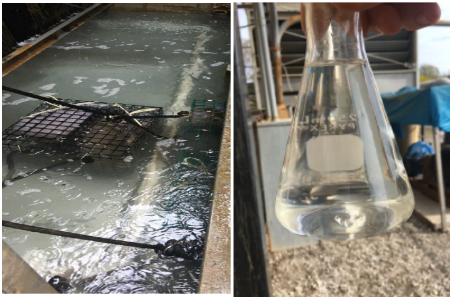
Fig. 2 After 1 month of ProMoss™ being added to treatment: Water clarity improved dramatically. Foaming minimal. No new organic contamination formation.
