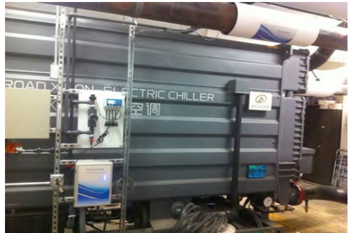
FlowMark Chemical-Free Electronic Water Treatment System with conductivity meter, probe and blow-down assembly.
