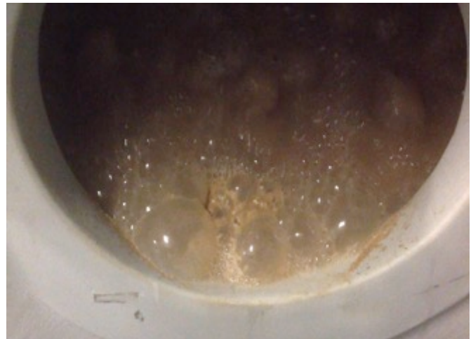
Sand filter during Air Scour treatment with Breakaway ® flush
