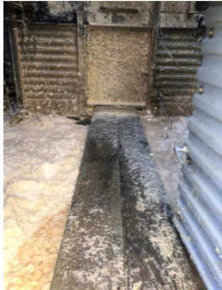
Fig. 1 Before ProMoss™: Water heavily contaminated with product from process systems and microbial growth. Thick organic contamination build up. High turbidity and heavy foaming.
