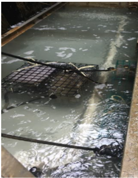
Fig. 2 After 1 month of ProMoss™ being added to treatment: Water clarity improved dramatically. Foaming minimal. No new organic contamination formation.
