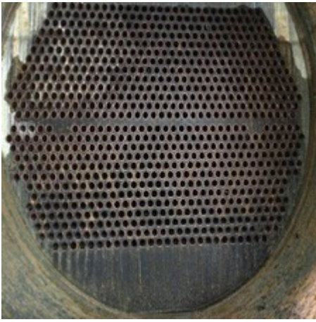
Figure 4. Chiller treated with ProMoss™ after opening with no cleaning
